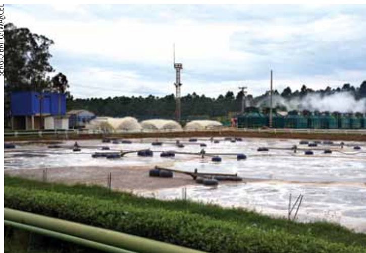
Lwarcel's waste treatment station. The adoption of practices aimed at using and reusing water sector by sector in a rational manner was the solution found to reduce the amount of water captured and effluent generated
