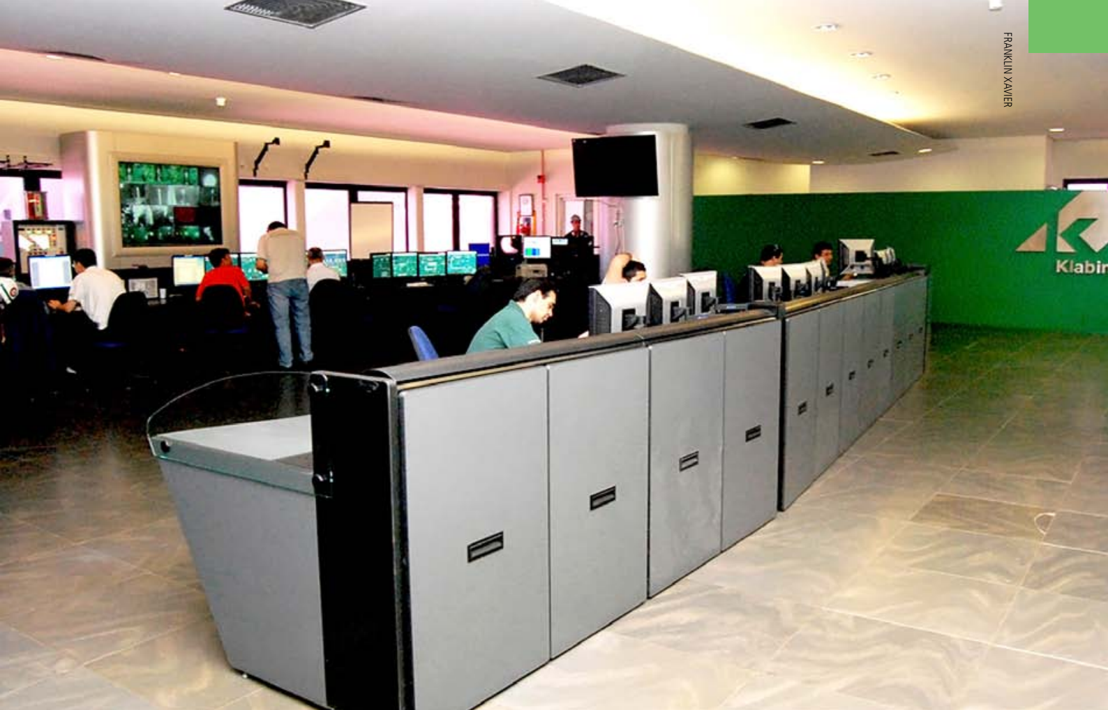
MP9 Control Room: integrating operational controls of a paper machine in a single environment is already done at Klabin
