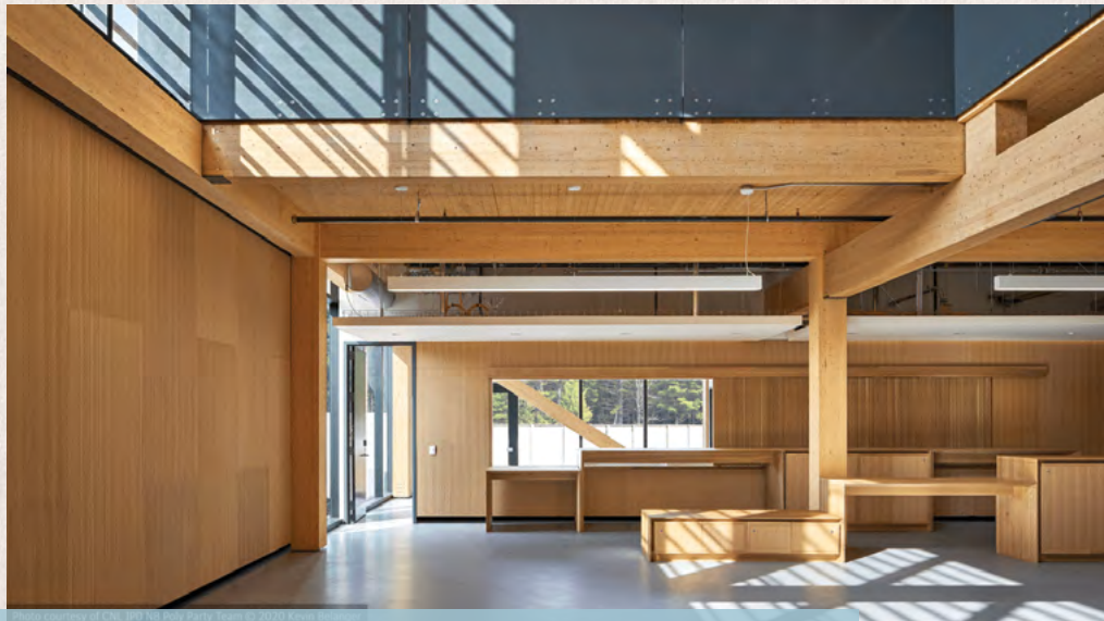
Mass timber project at Chalk River Laboratories, Ontario, Canada. Credit: Nordic Structures
