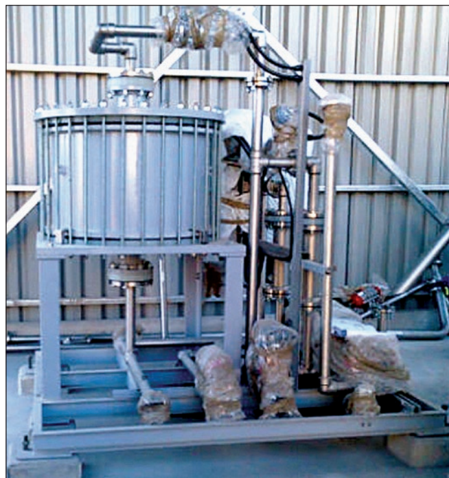
Figure 4. Pre-assembled and tested functional modules at Arauco Constitución mill
