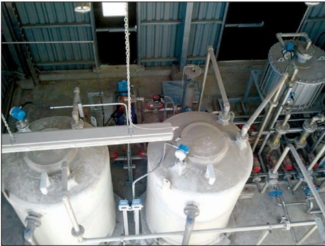
Figure 6. Installation at Arauco Constitución mill
