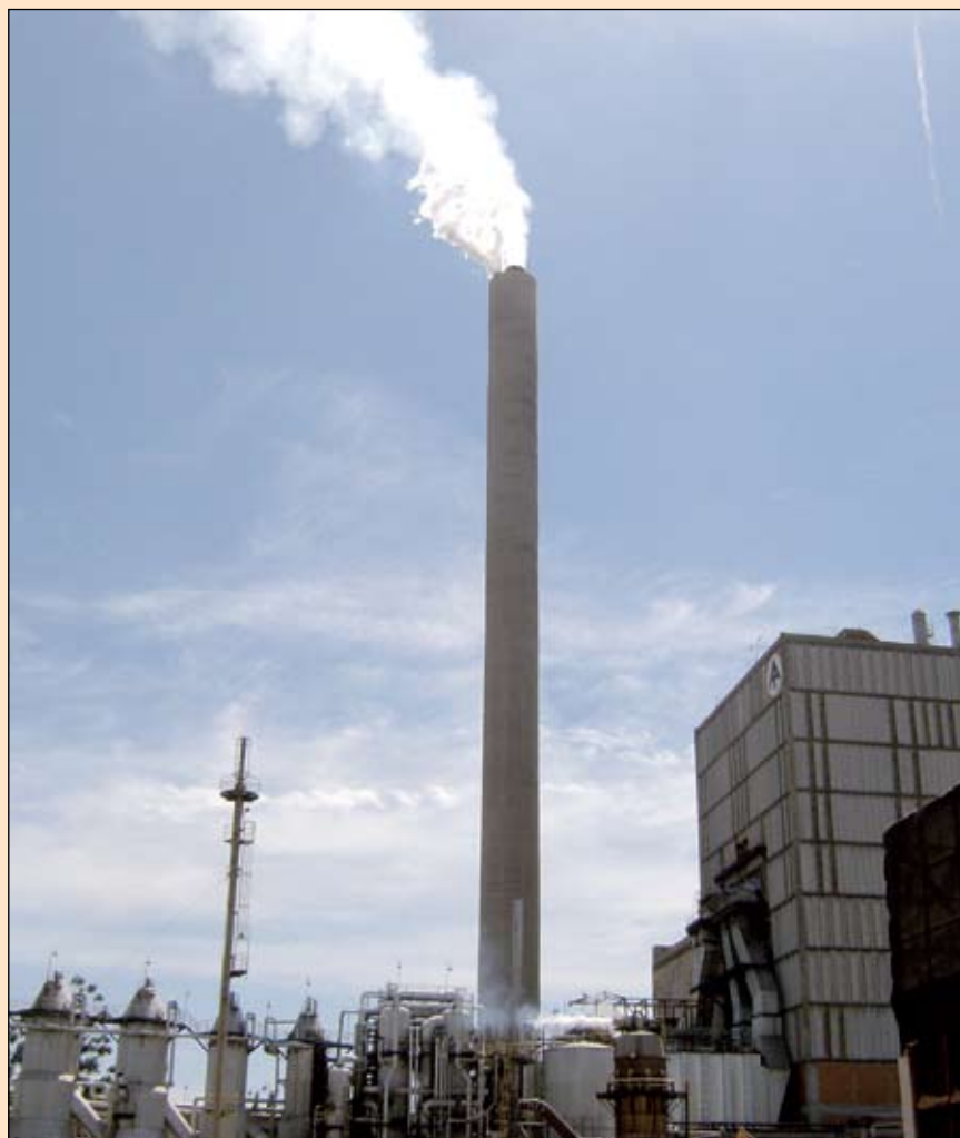
Reduce the emission of particulate material is the main difficulty for older mills
