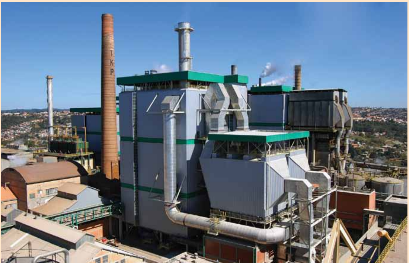
Klabin's new biomass boiler can use all the forest waste from the region where the mill is installed
