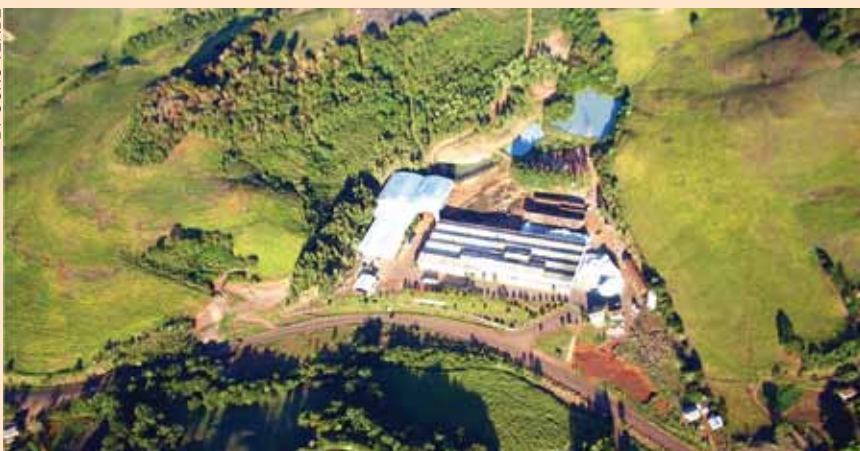
Ouro Verde plant in Brazil
